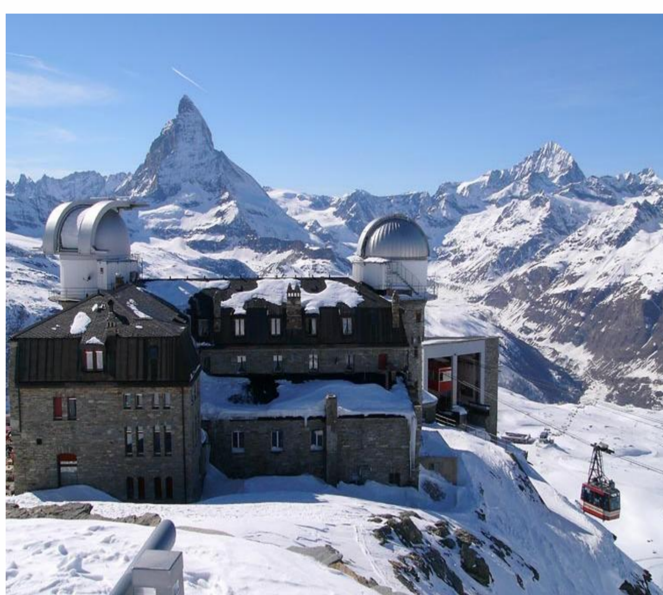
Figure 1: The Kulmhotel Gornergrat was opened in 1910, above the top-station of the Gornergratbahn. In the year 1985 two astronomic observatories were added to the northern and southern towers, built on permafrost. To the right, a funicular constructed in 1957 leads to Hochtälli (3286 m) and Stockhorn (3407 m). Ice-filled bedrock joints at the construction sites prove the existence of permafrost, there. The prominent peak of Matterhorn (4478 m) is seen in the background.
