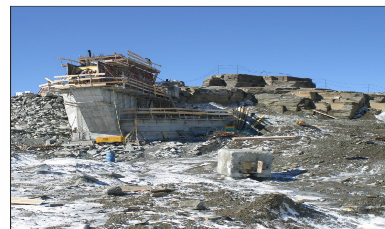
Figure 7: Same location as above, during construction in 2003.
