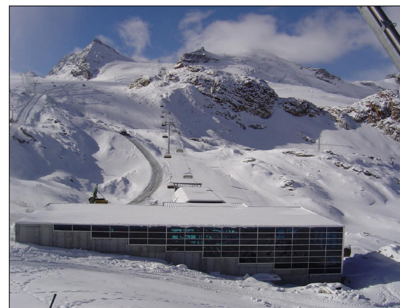
Figure 8: The new Furggsattel (6 persons) glacier chairlift leads from Trockener Steg (2929 m a.s.l.) to the crest of Furggsattel at 3351 m a.s.l. It guarantees year-round skiing, as the ski-run leads mainly over the glacier Oberer Theodul. Twelve masts out of 17 have been constructed on the glacier with special devices for adjustment to the glacier movement. The building in the foreground receives the passengers from Furgg (2432 m).
