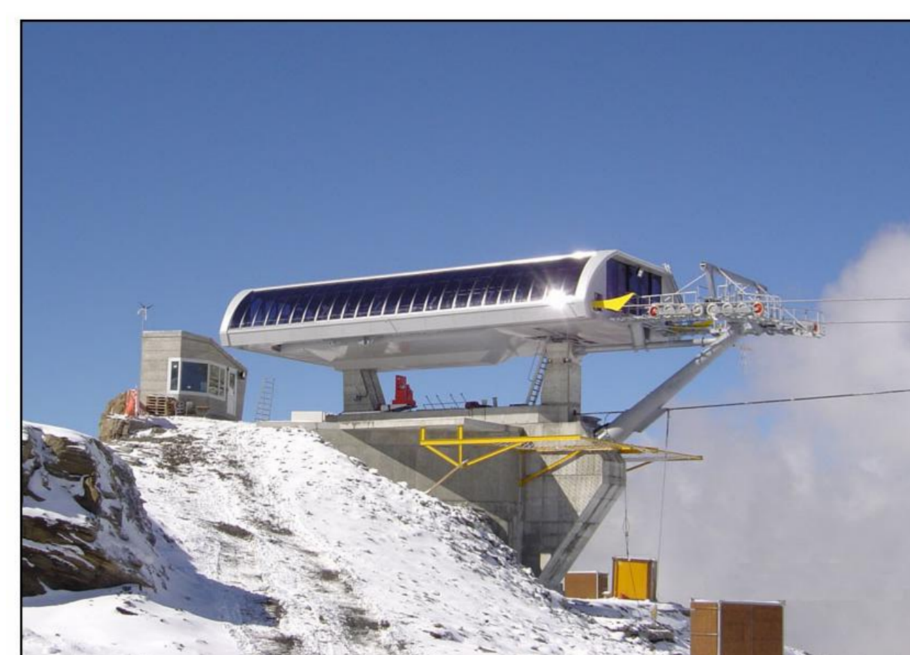
Figure 6: The top station Furggsattel is anchored deep into the perennally frozen bedrock. It is located at the mountain crest (background) that also marks the Swiss-Italian border.
