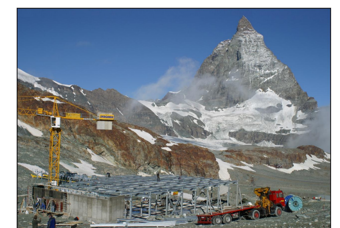
Figure 9: The station Trockener Steg during construction phase in summer 2003 (cp. Figure 8).
